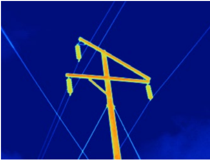
Figure 7: High voltage power pole, captured with a TiX560 camera and standard lens.
