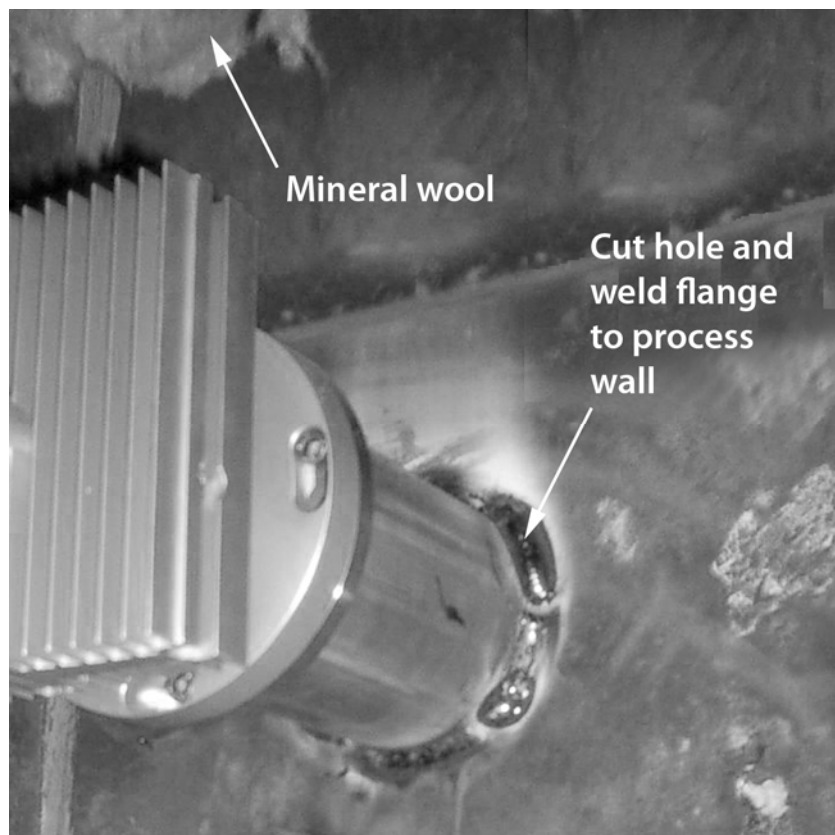
Figure 82 Cooling Set Installation
