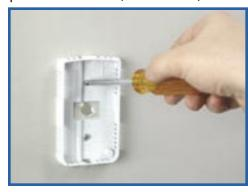
2) Connect circuit board to wall plate.
