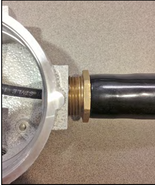
Figure 17: Torquing the Cable Gland
