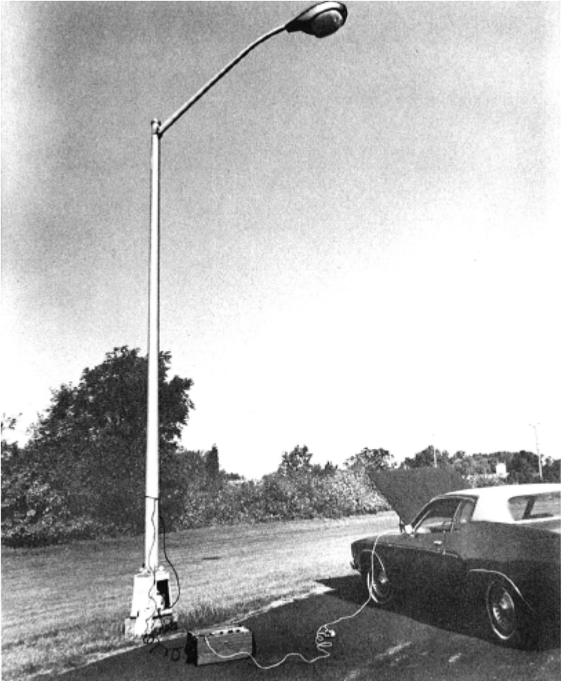
Figure 5: Testing Parking Lot Lighting; the Test Set Shown is Operating from an Inverter.
