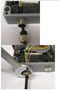
Feed the transmitter cable through the sleeve and tighten the cable gland.
