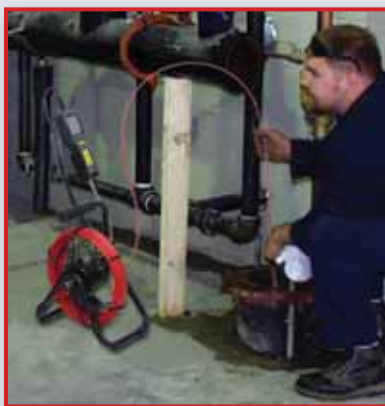
Monitoring the clearing of a clogged sewer drain
