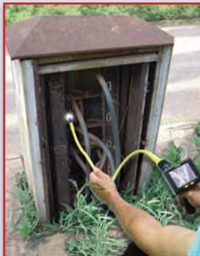
The DCS400-PE makes it safe to inspect structures, like this open utility box on the street that may have been tampered with
