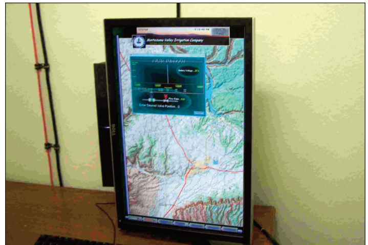
Figure 3: Flow control and measurement is implemented via a wireless supervisory control and data acquisition (SCADA) system. The SCADA system consists of a telemetry receiver and master control center in the main office connected to field equipment via a wireless data link.
