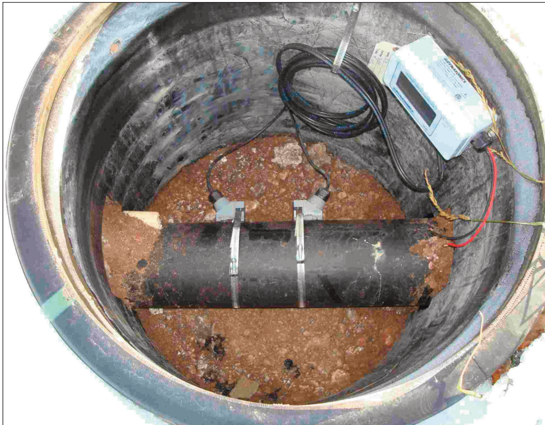
Figure 2: The transit time flow meters use two transducers mounted on the outside of the pipe, both of which function as an ultrasonic transmitter and receiver.
