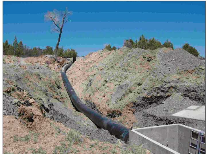
Figure 1: Open ditch irrigation canals were replaced with a closed poly pipe water distribution system. The piping system saves water by reducing evaporation, cutting seepage and eliminating end of channel water losses.
